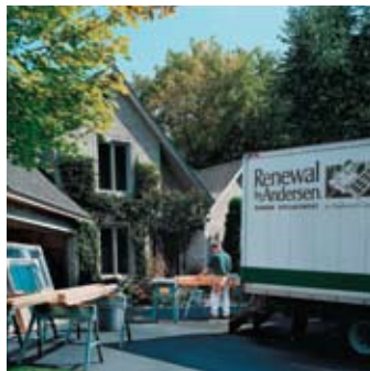
Our installation professionals demonstrate the utmost respect for your home throughout the installation process and leave your home and yard clean and tidy.
